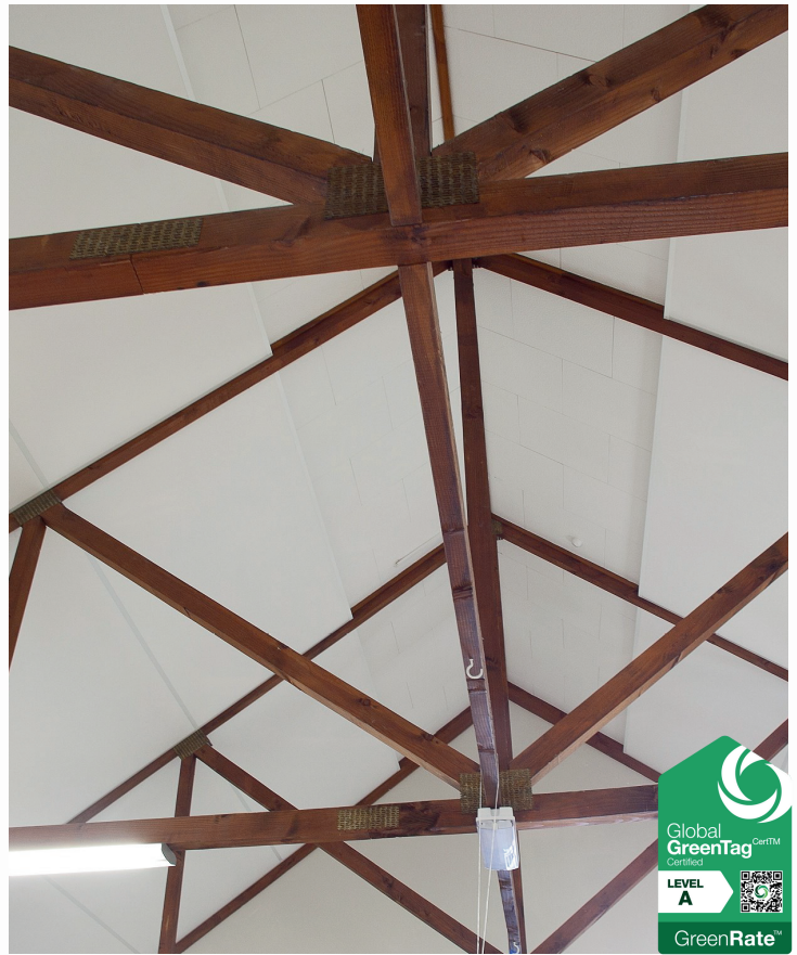
Photo: Triton 50, 2400 x 1200 panels direct fixed over plasterboard lining in retro fit of existing classroom.
