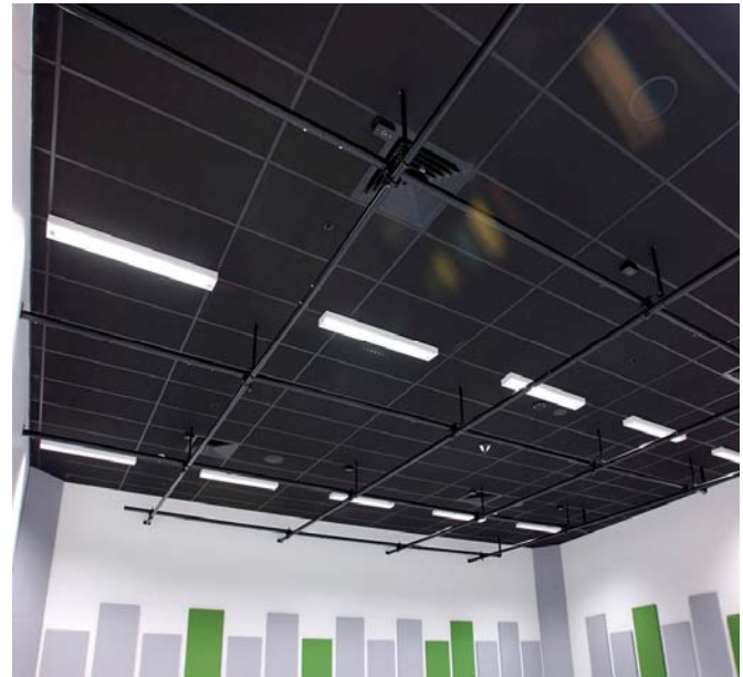
Hobsonville Point Secondary School, Triton 25 with black Sonatex facing
