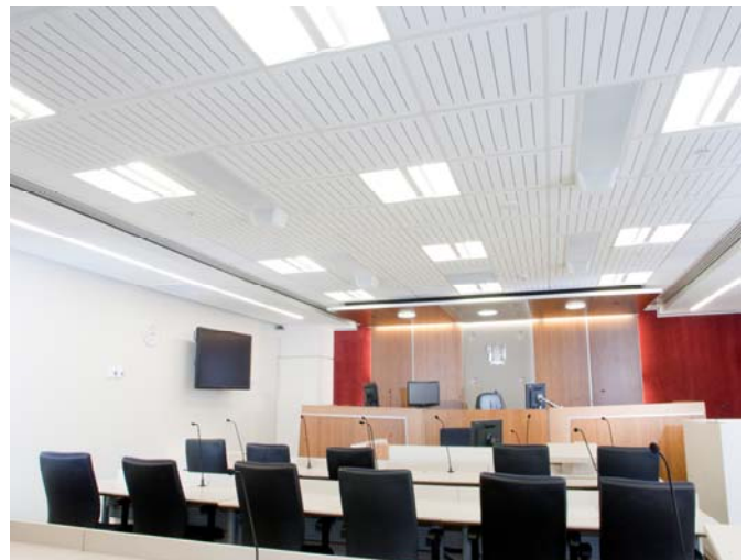
Auckland District Court—Triton 50 with 7 x 500 slot perforated white on grey facing
