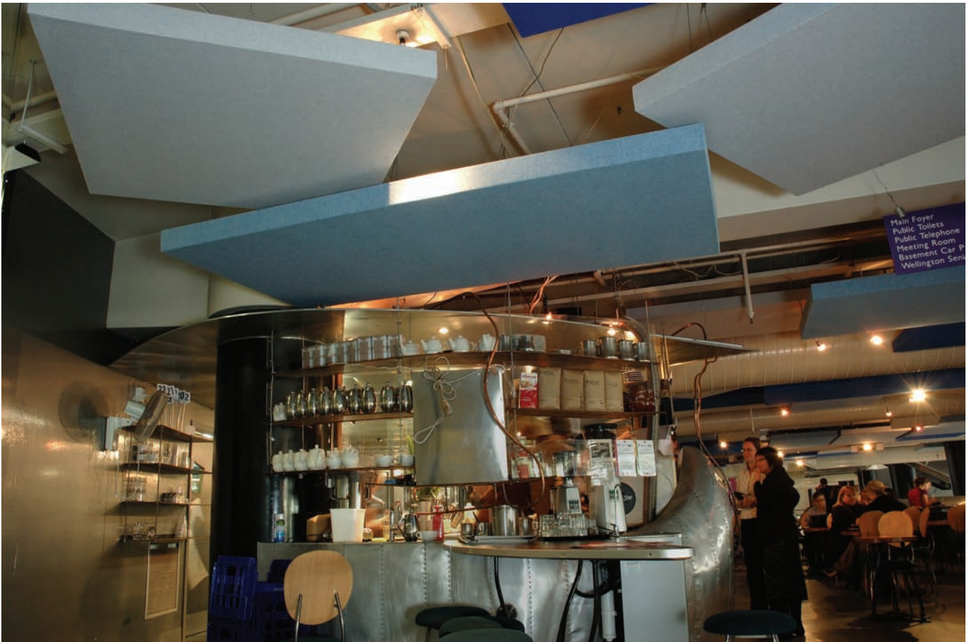
Top: Asona Fabwall 100 ceiling cloud panels
