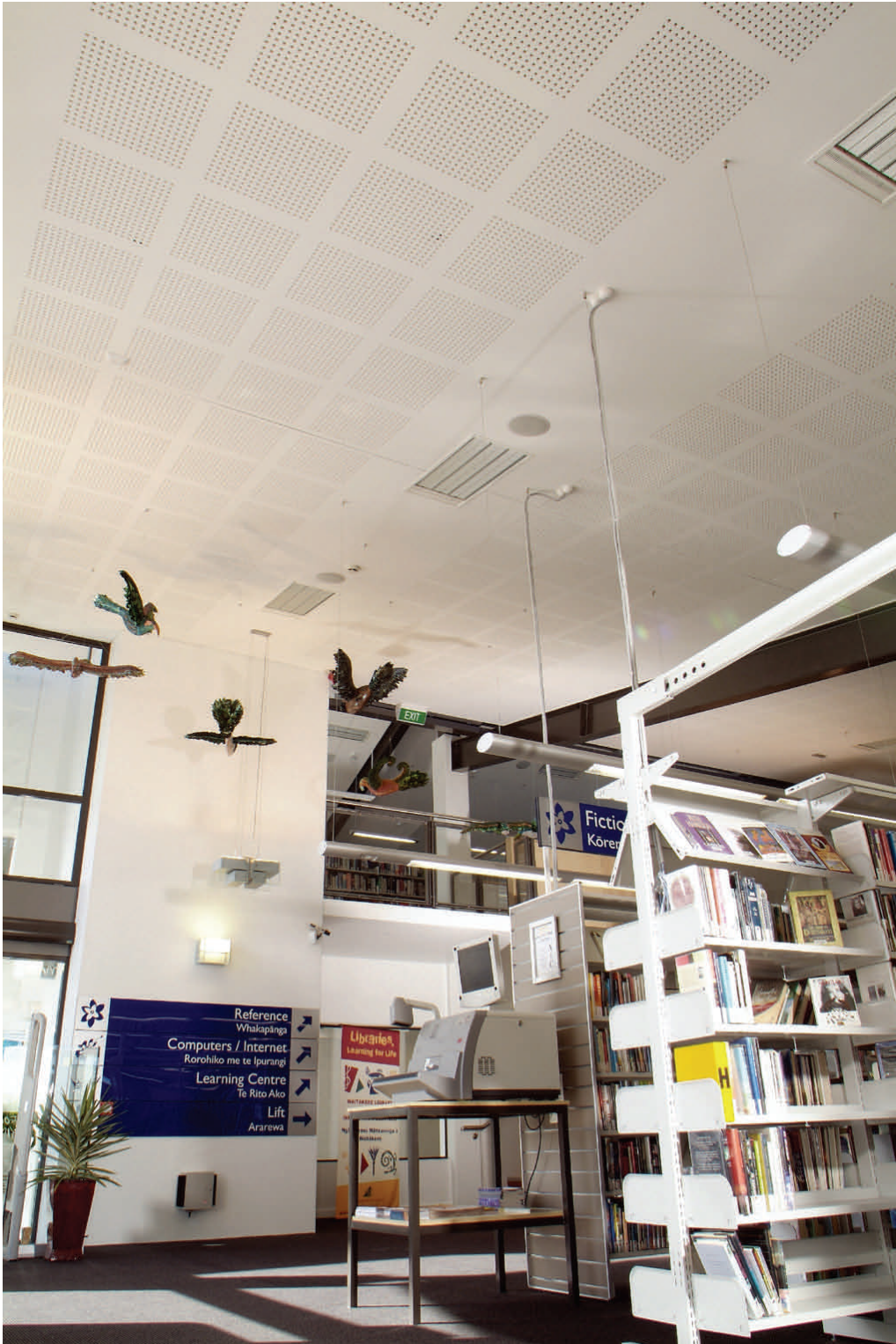
Above: Danoline Designpanel 1200 perforated plasterboard acoustic ceiling system Perforation Q2F 12 x 12 mm square perforation in 475 x 475 mm clusters 2400 x 1200 x 13 mm sheets screw fixed to metal furring suspension at 300 mm centres. Flush stopped to level 4 and painted with fine nap roll
