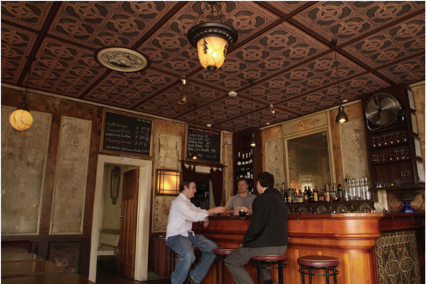
Top: Asona Triton Image™ digitally printed bespoke composite soft absorber ceiling panels with timber moulding cover batten.
