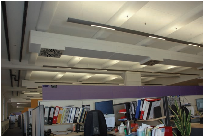
Top: Asona Triton 25, custom size 1650 x 1200 mm panels on TFX tissue faced grid help express the exposed beams
