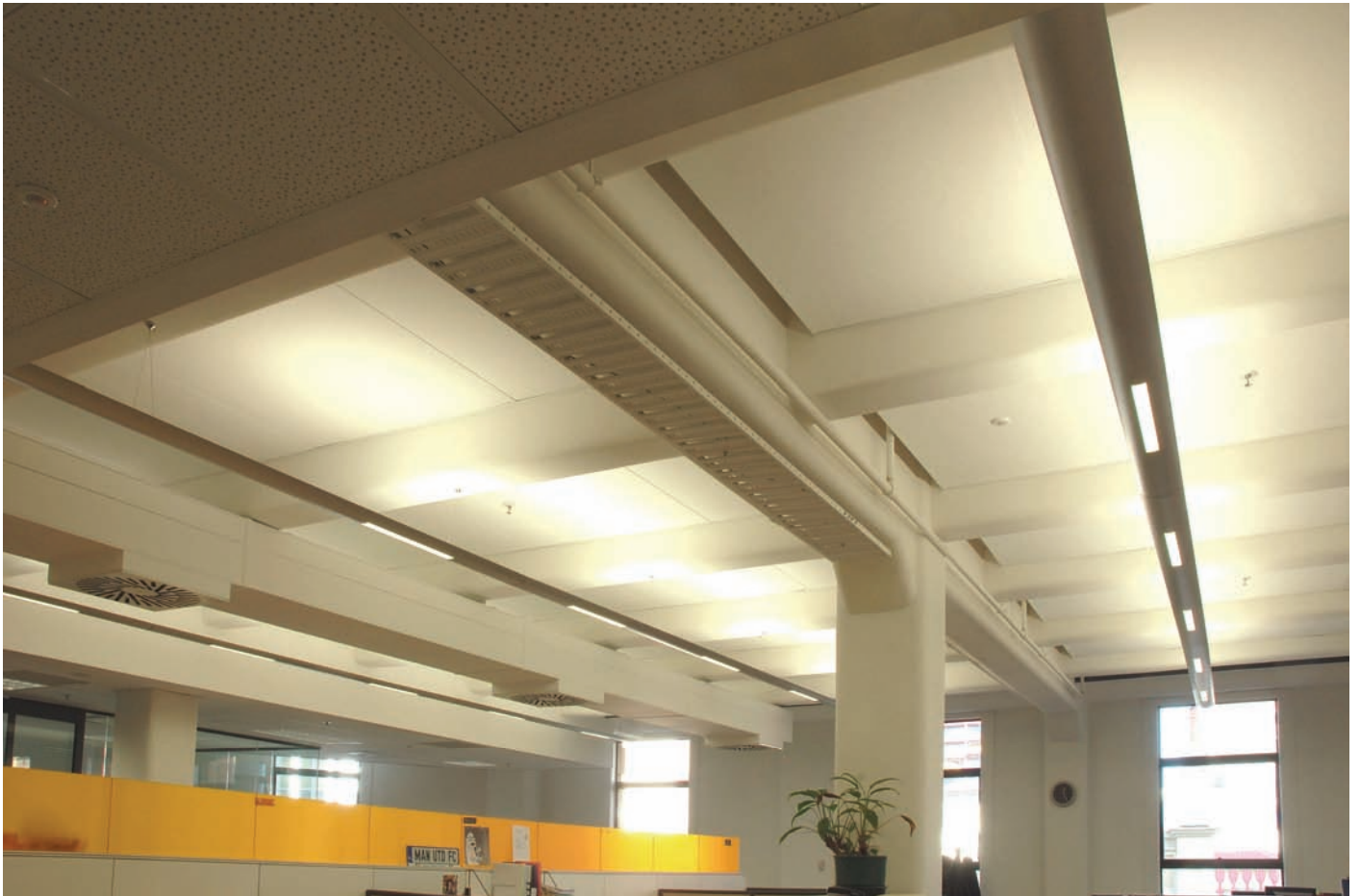
Top: Asona Triton 25, custom size 1650 x 1200 mm panels on TFX tissue faced grid help express the exposed beams
