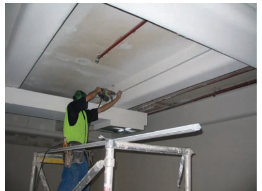
Top: Asona Triton 25, custom size 1650 x 1200 mm panels on TFX tissue faced grid help express the exposed beams
