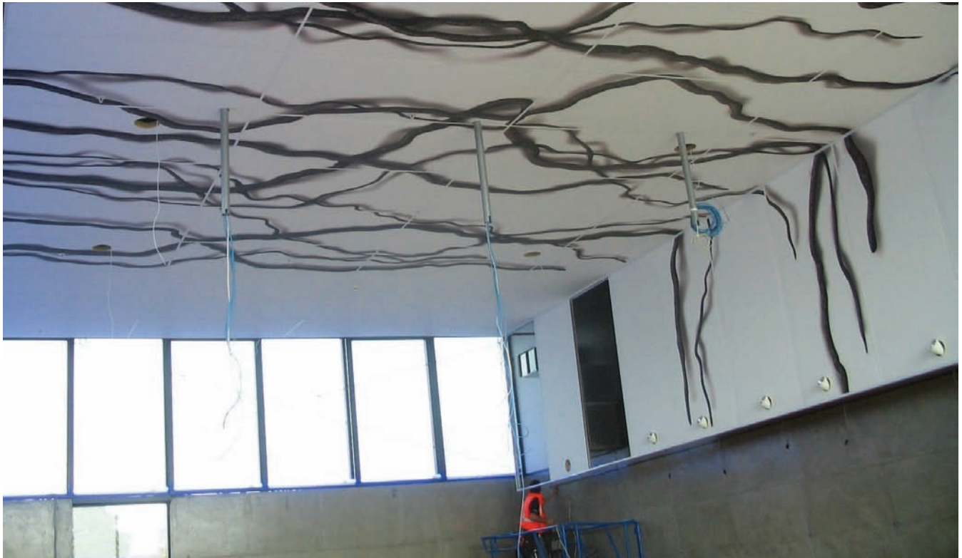
Wintec Library, Hamilton. Triton Image 2400 x 1200 x 50 mm panels on TFX tissue faced grid. Panels printed with a bush vine image running across ceiling and down the bulk head
